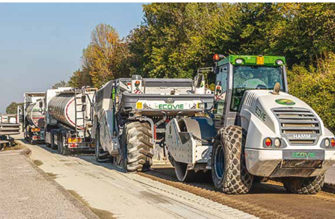
5. Cantiere Ecovie Srl (photo credit: Ecovie Srl)
