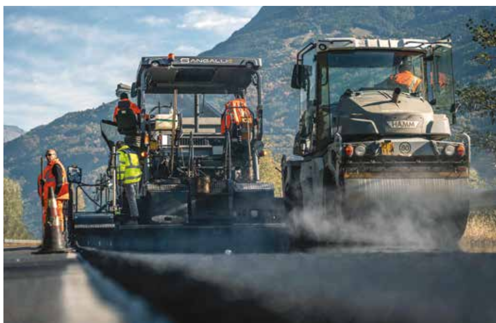
3. Cantiere Sangalli SpA (photo credit: Sangalli SpA)
